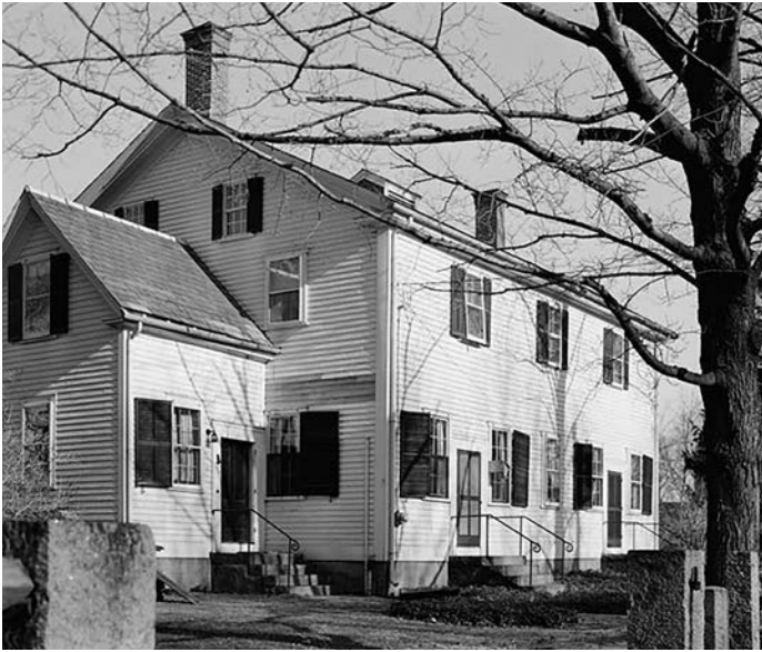
The 1791 meetinghouse at Harvard, Massachusetts. It was relocated in 1854, given a gable roof, and stairwells to the second floor outside of the original footprint of the building. Photograph by Jack E. Boucher. Historic American Buildings Survey, Library of Congress, Prints and Photographs Division, HABS MASS,14-HARV,8-2 (April 22, 1963)
