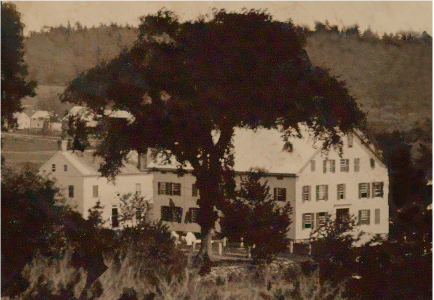
Fig. 5. Detail of Harvard South Family Wash House and Dwelling House.
