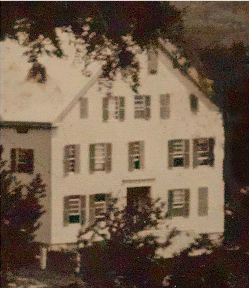
Fig. 6. Detail of Harvard South Family Dwelling House facade.
